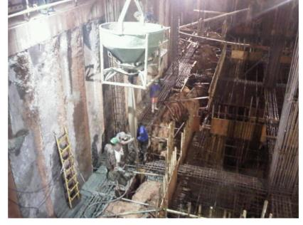
design for the concrete (subject to area was 350kg/m3 to 450 kg/m3).
